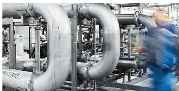
Production at the BMW plant in Steyr, Austria, has completely closed the water cycle and is thus wastewater-free.
