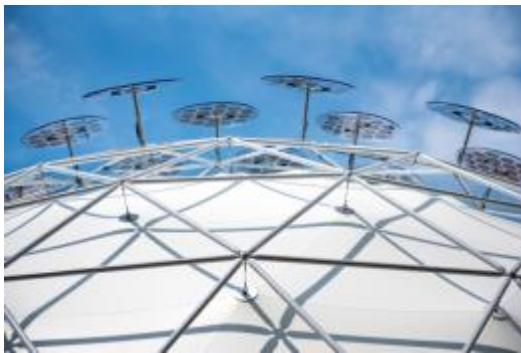
Picture 1: Close-up of the OPV solar umbrellas on the bearing structure of the "Climate Pavilion"
