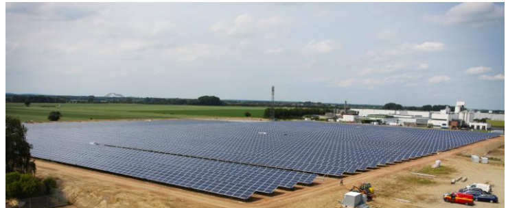
[Caption] On the grounds of the former sugar factory in Gross Munzel, AS Solar has built the largest solar park in the Hannover metro area. (File: as_solar_gross_munzel.jpg)
