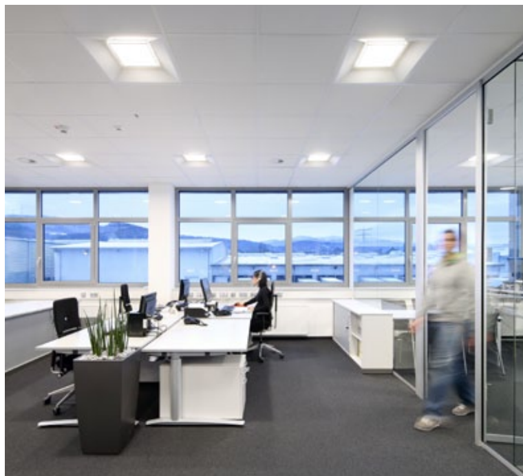
B2 | The LED lighting solution in the offices sets new standards for efficient high-quality task lighting. As a special solution, the Crayon LED downlight has been mounted flush with the ceiling, thus ensuring flexible room use.
