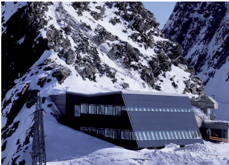
PV installation at „Matterhorn Glacier Paradise“
