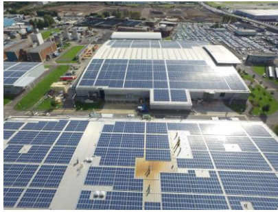
Photo 01: The new PV power plant at Rolls-Royce factory rooftops with nominal power of 3.42 MWp
