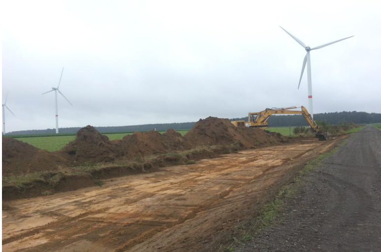
Topsoil removal for road and crane hard standings
