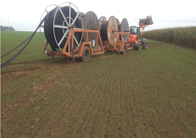
Cable installation by means of cable plow and drilling
