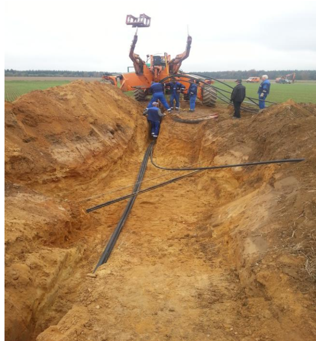
Cable installation by means of cable plow and drilling
