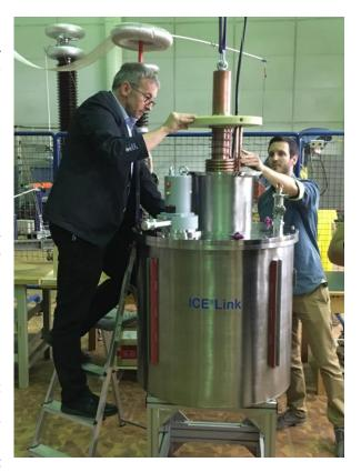
includes the installation of a 25 meters superconducting busbar system which is feeding a real operative industrial production unit with 20 kA direct current. Endurance tests of all components, including the refrigeration system, will thus take place under industrial working load conditions.
