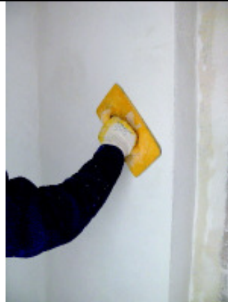
4. Rub-off of the surface of INTRASIT RZ2 File name: S03Bild4 Photo: Heinrich Hahne GmbH & Co. KG
