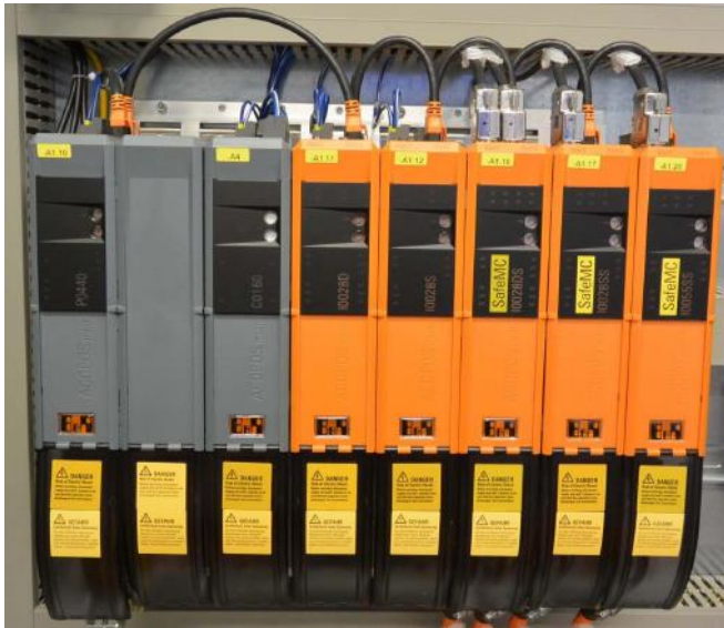
New AcoposMulti servo technology from B&R for the SMART - DM 402 dispensing cell with built-in safety technology
