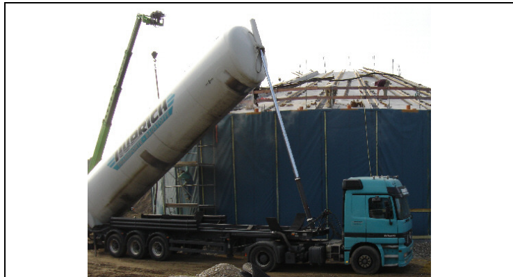
Preparatory work for the blowing-in of the insulation of the thermal energy storage silo in Munich.
