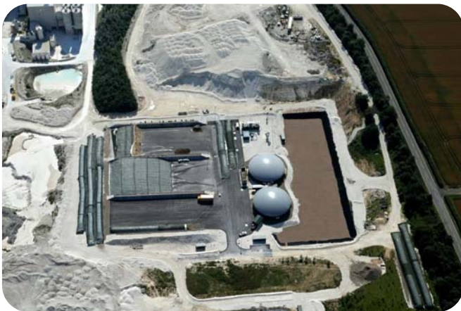
Picture 2: Aerial view Melton Ross
