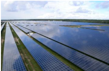
Picture Caption 01: With an output of nearly 70 MWp, Alt Daber near Wittstock is Europe's largest thin-film ground-mounted solar power plant
