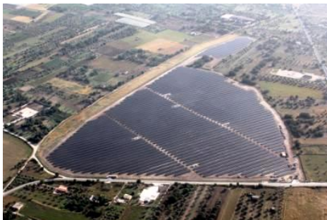
Picture Caption 02: BELECTRIC has constructed eight ground-mounted solar power plants in Italy with a nominal output of 42MWp. The solar power plant ‚Librandello‘ saves 8,100 tons of CO 2 per year.
