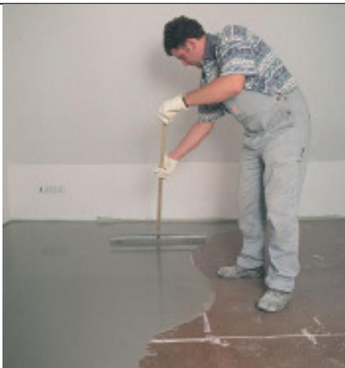
PCI Periplan Extra light is fiber reinforced, that flows easily and hardens quickly. Properties that pay off, particularly with renovation and upgrading work.
