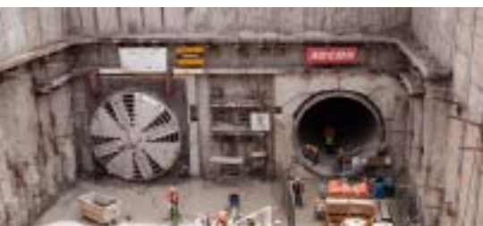
U-Bahn-Bau in Toronto Building the subway in Toronto
