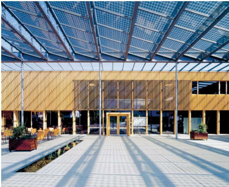
Room 2 Ecological balancing
