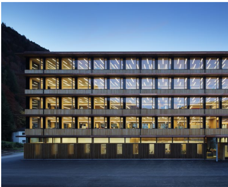
Room 3 A different construction phase
