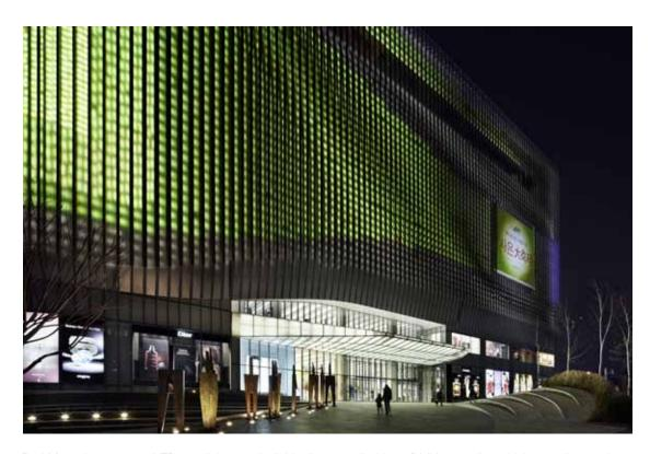
B2 I More than 22,000 LED spotlights are individually controlled by a DMX controller which coordinates them to produce unique façade lighting. Zumtobel realised the lighting solution project specifically in accordance with ag Licht's lighting design.
